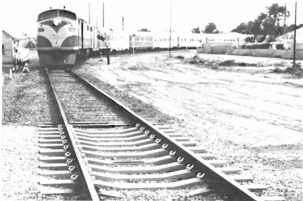
An ANR passenger train about to pass over a section of track laid on 10 "GOLDEN" concrete sleepers, including the one-millionth supplied to ANR.
