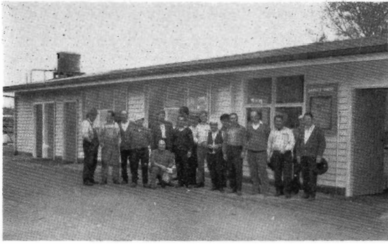
Some of the 31 men employed at the depot. Jobs include gantry and mobile crane drivers, floormen, a tractor driver, oil and brass furnacemen and office staff.
