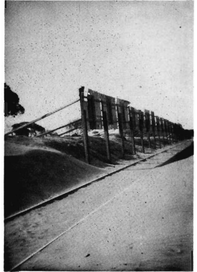
At Sea Lake the effects of the length of chute erected by Mr George and his gang can be seen. Sand has been kept off the track in front of the barrier, but in the foreground, where chute was still to go up, sand surrounds the line. That was in 1938 — a dry year.
