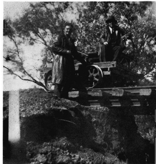
Mr George (left) was District Engineer at Bendigo when this photo was taken of him with his roadmaster, Mr M. Hogan. The two men had just inspected a new bridge built by the railways after the Charlton floods in 1939.
