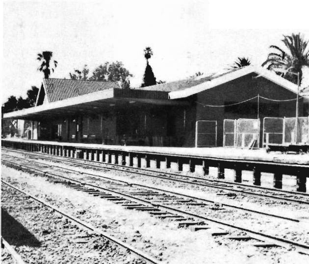
Mildura's new station building. Not one outside wall of the old station remains.
